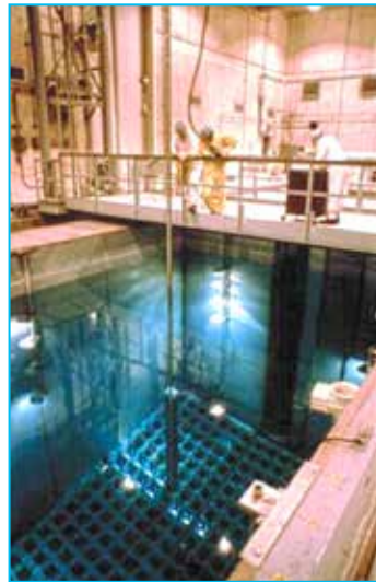
Spent Fuel Pool
