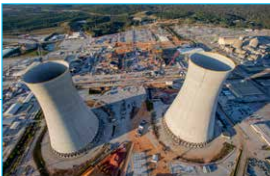
New units at Plant Vogtle
