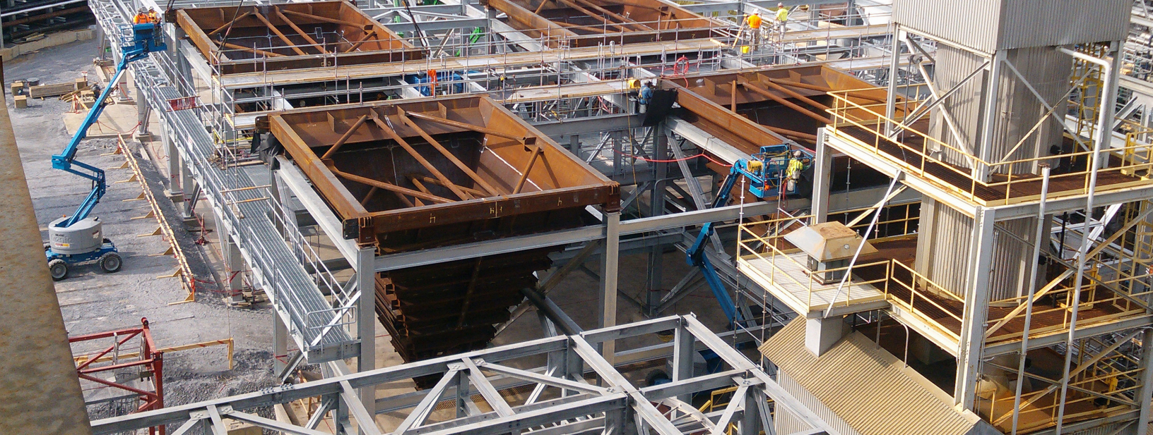
Construction of a baghouse at Alabama Power's Plant Gaston
