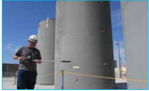
A radiation protection worker does routine inspection of the dry cask storage area inside the secure area of Plant Farley.
