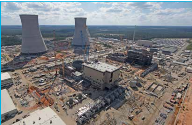
New units at Plant Vogtle
