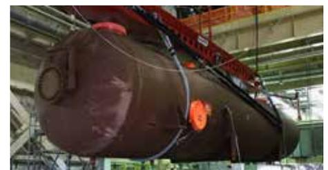
One of two massive 83.5-ton feedwater heaters replaced during the outage.
