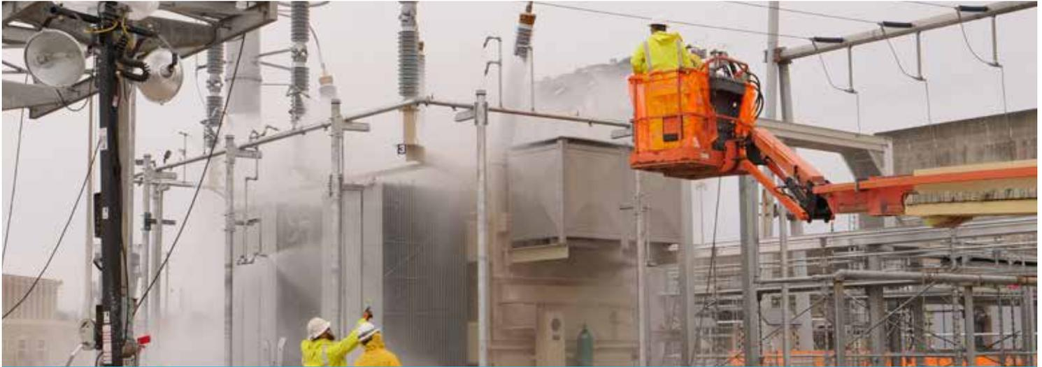
Fire suppression testing was completed before the new transformer was put into service.
