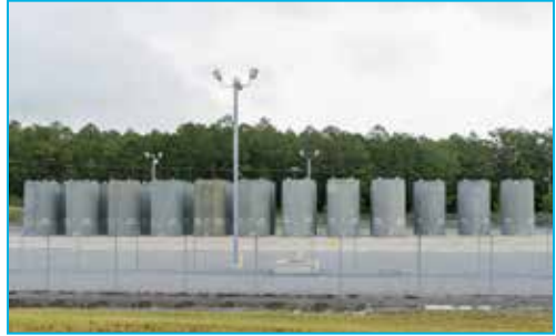
Currently, used fuel is being stored in dry cask storage as well as in the spent fuel pool at Plant Hatch.
