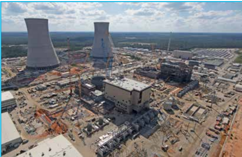
New units at Plant Vogtle
