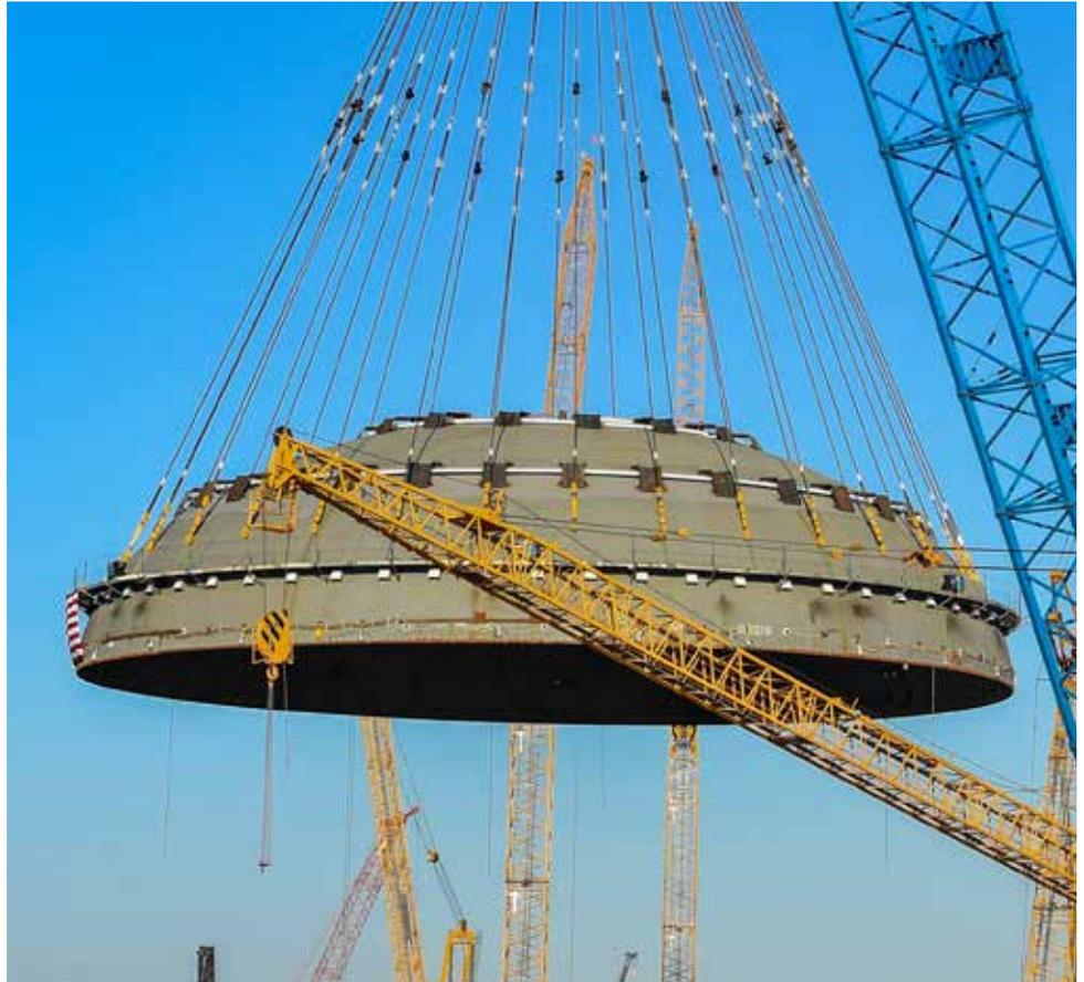
*The placement of the Unit 3 containment vessel top head marks a significant milestone in the Vogtle 3 & 4 project.*
