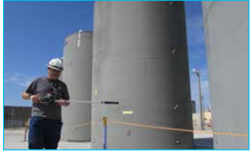
A radiation protection worker does routine inspection of the dry cask storage area inside the secure area of Plant Vogtle.
