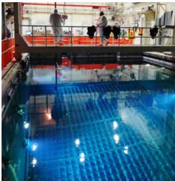
Spent fuel pool
