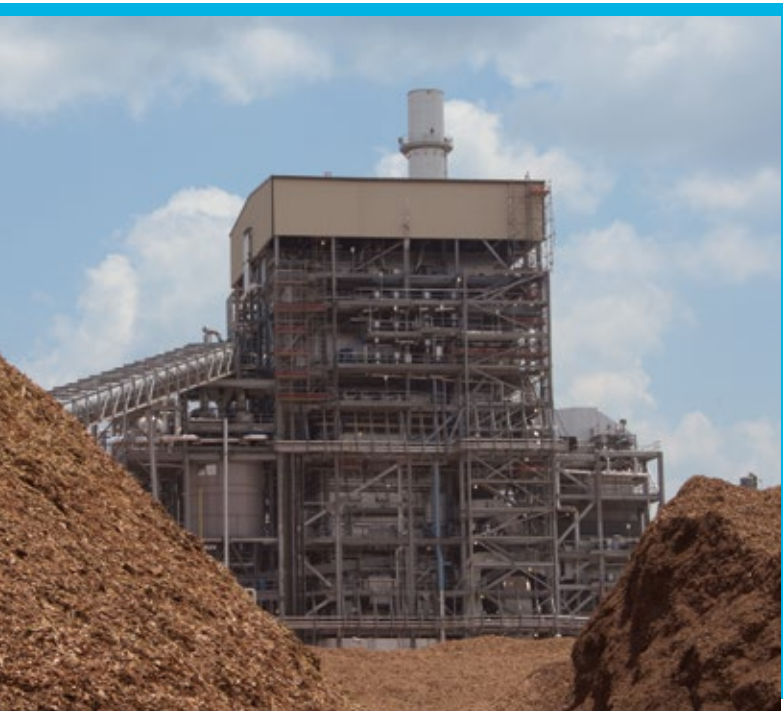
Nacogdoches Generating Facility
